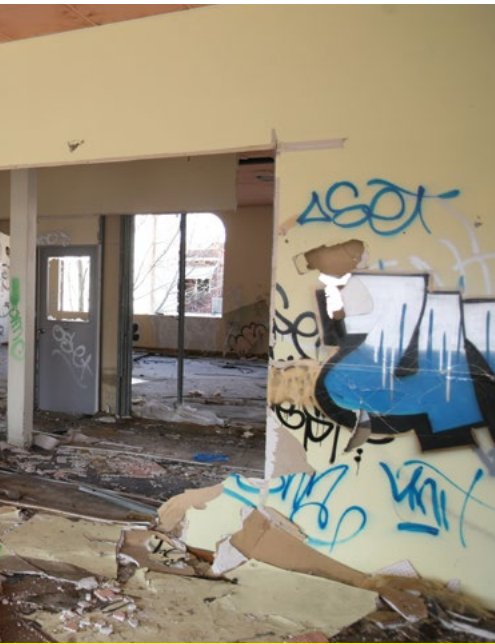
Removal of interior ceiling tiles by vandals will allow rapid interior vertical fire spread through a building; a metal truss roof [vulnerable to early collapse] is located above the ceiling line
