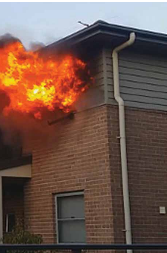
A window located on southern side of the building, acts as an inlet opening, located on the upwind side of the fire. Note, flames are not venting outwards. Also, compare fire activity with the vent outlet. Both windows are fitted to the same fire compartment. The defensive attack stream directed through this window reduced fire intensity within seconds. Picture supplied courtesy Mrs Amy Johnson
