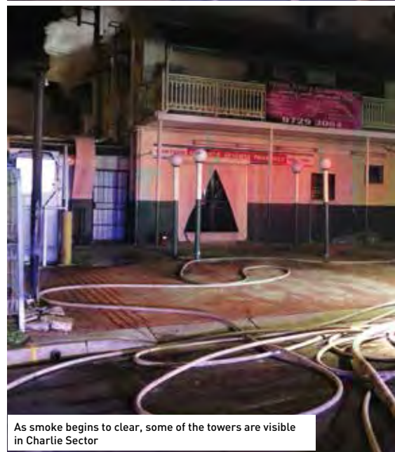
The fire building from Sector Alpha. The mobile phone towers are completely obscured by smoke
