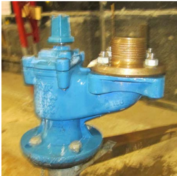
Figure A-3: Ball valve hydrant
