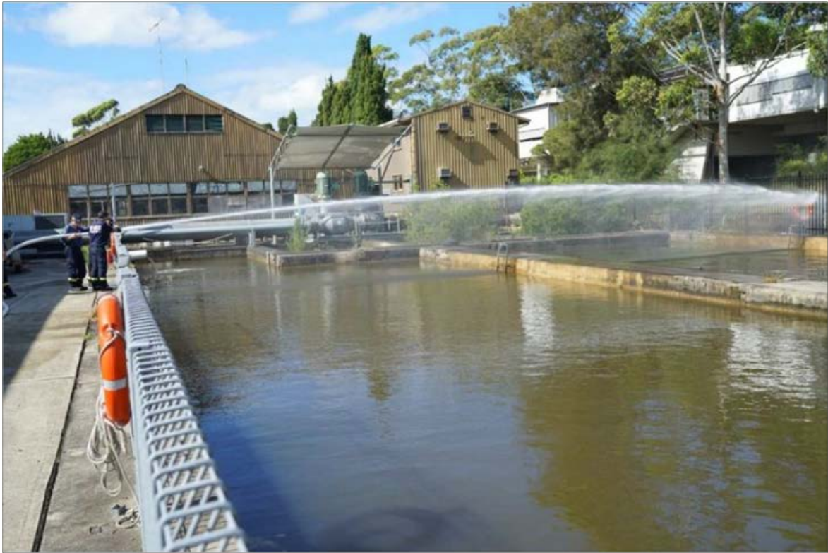
Photograph: 10 l/s water stream issuing from an FRNSW Ø65mm Akron branch via a single Ø64mm x 30m of lay-flat canvas hose
