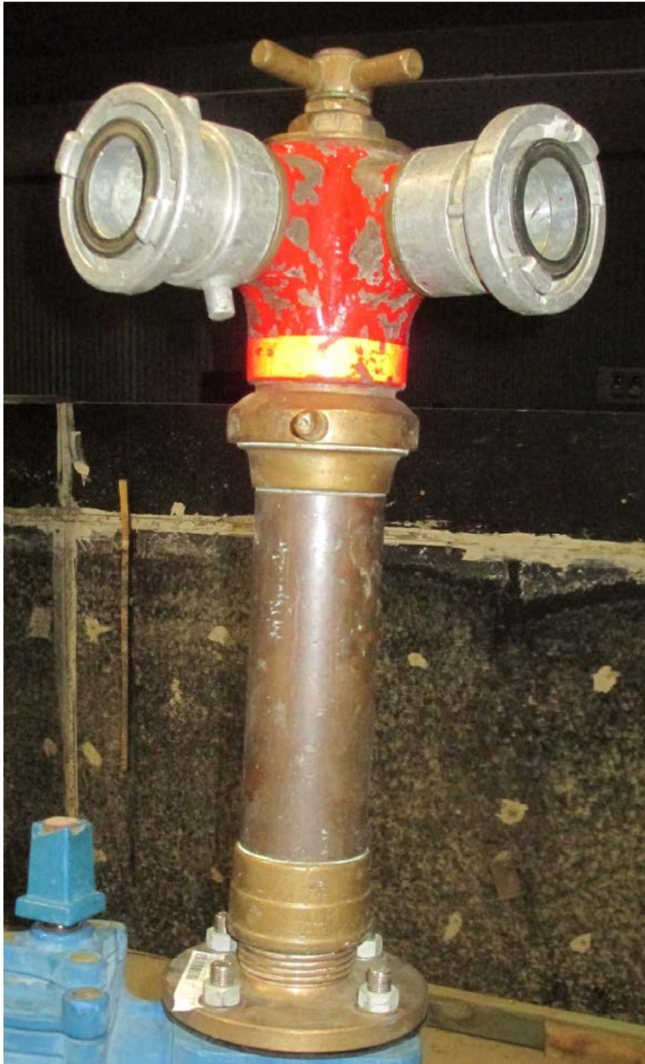
Figure A-7: Double delivery with Storz outlets
