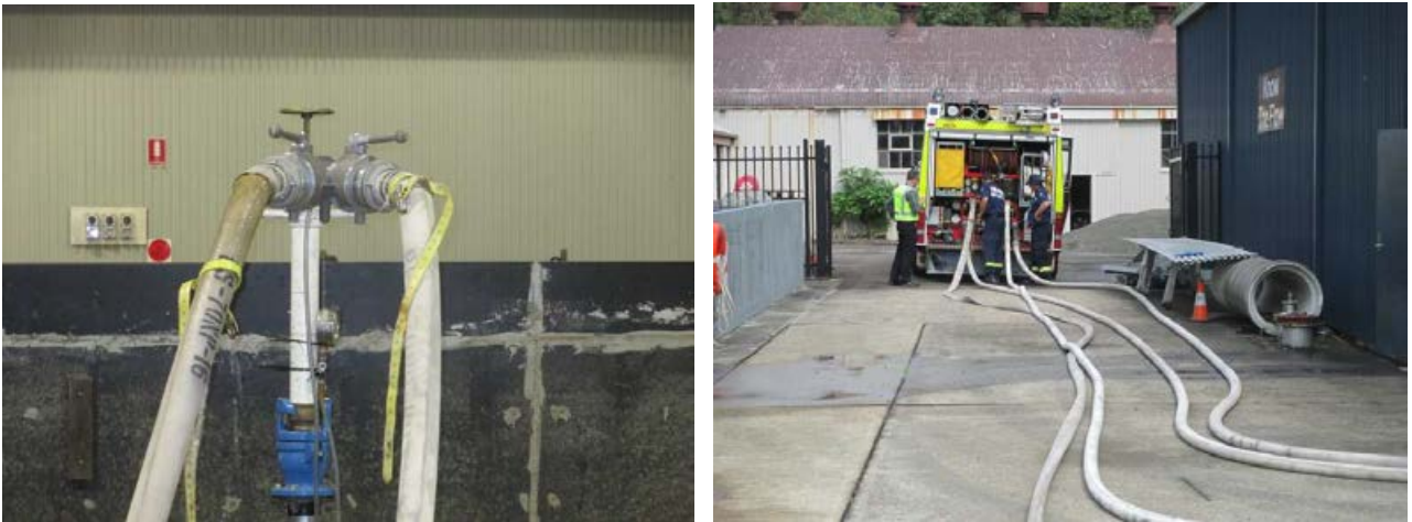
Figure 2-3: Hydrant supply to fire-fighting pumping appliance
