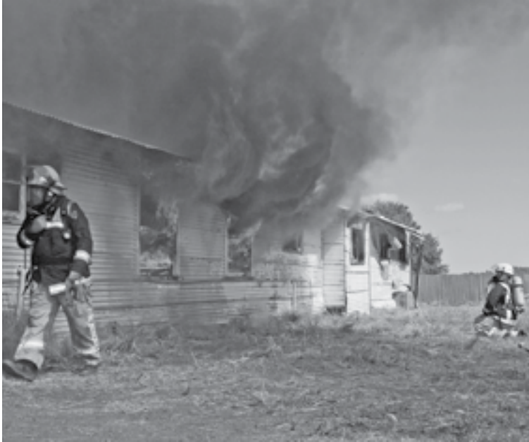
FRNSW burns a donated building at Parkes to conduct joint fire investigation training
