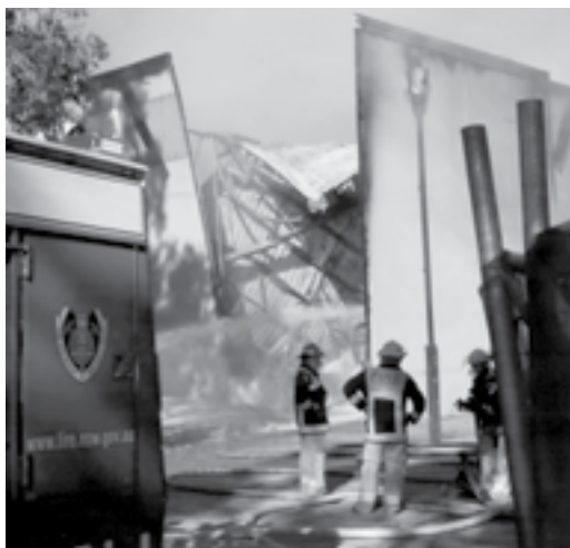
Left: Fire officers inspecting concrete tilt slab collapse following fire in retail superstore at Penrith (Photo courtesy Kernin Lambert) Right: Fighting a fire in a tyre factory at Campbelltown
