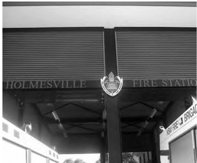
The new Holmesville Fire Station is improving fire and rescue services in Newcastle
