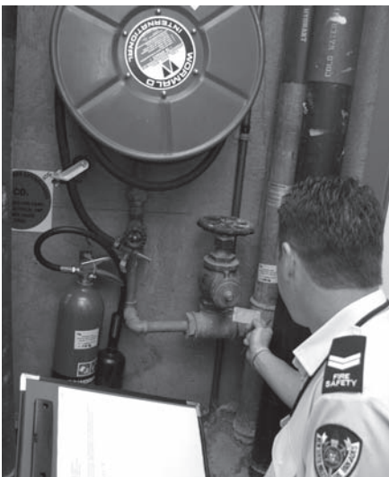
Inspection of fire protection equipment in commercial building
