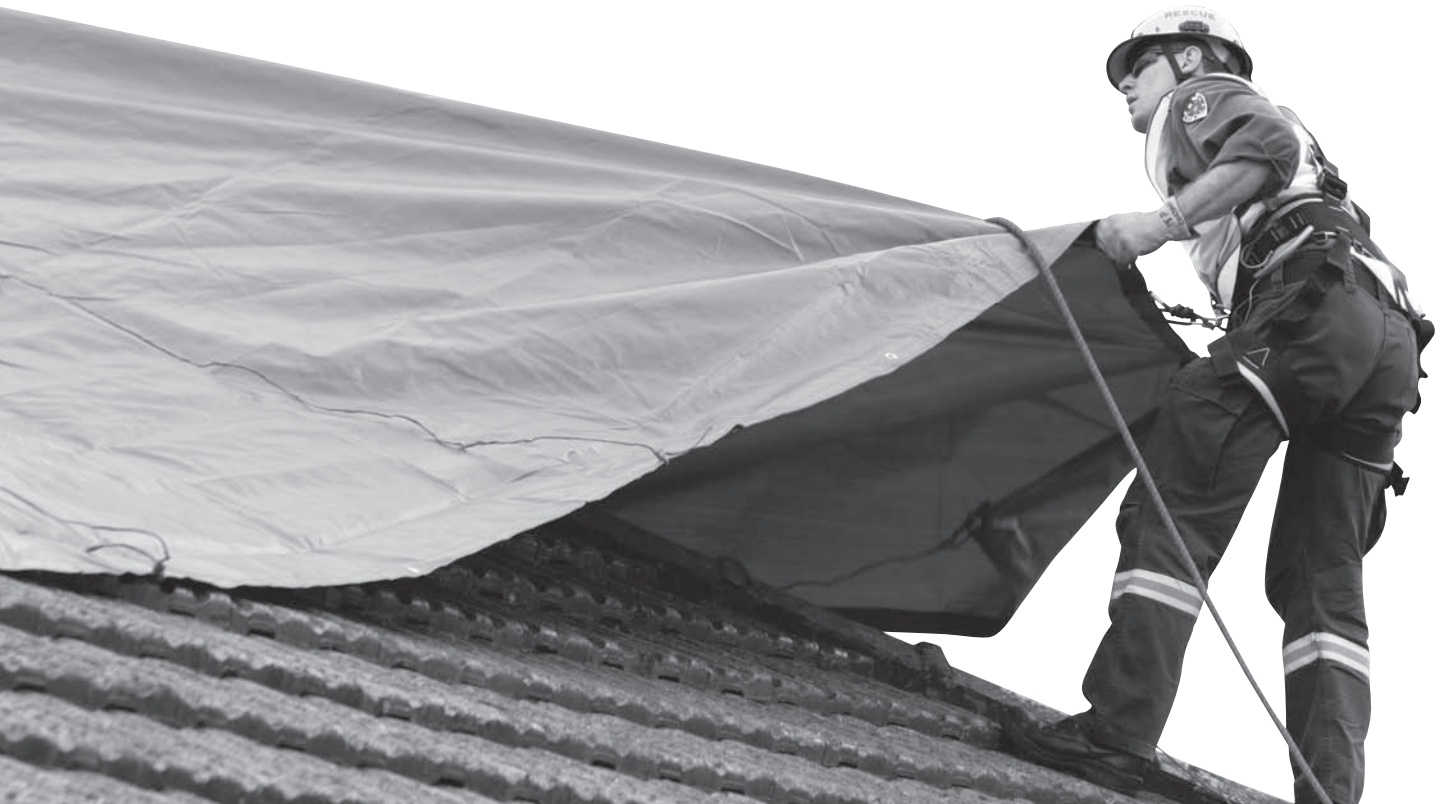
Covering storm-damaged roof with tarpaulin
