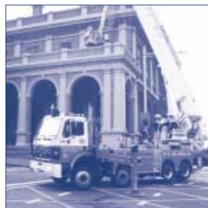
Firefighters extinguish a fire in the historic Sydney Supreme Court building.
