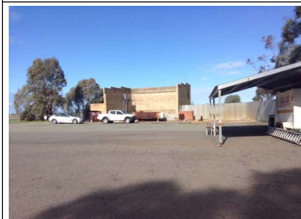
▲ Photograph 3: Centre of hardstand area looking south. Bricked training area and former bunded foam training area visible.
