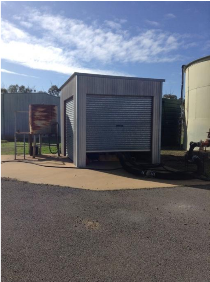
Appendix 17 – former fuel storage
