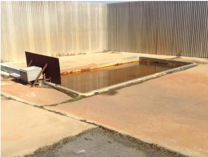
Appendix 5 – where AFFF training was. Pit lit by gas and hoses used to extinguish. Fence wasn't always there
