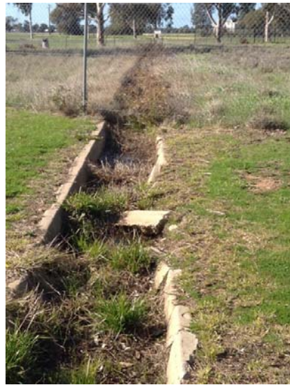
▲ Photograph 16: Drainage line leading off site (north of eastern boundary)
