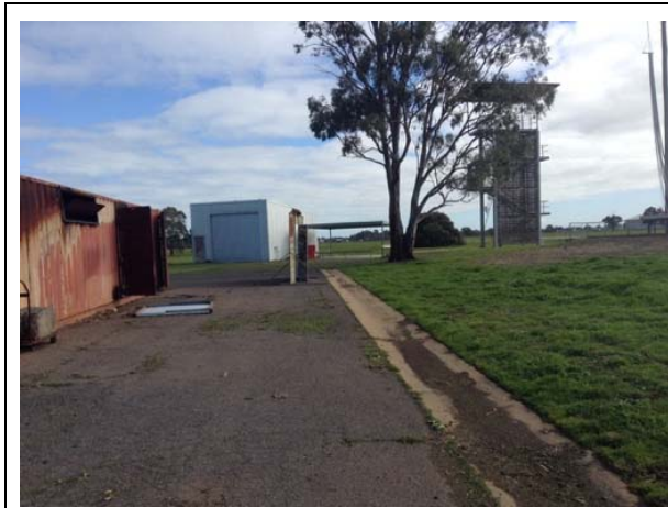
▲ Photograph 1: Shipping container used for fire training. Drainage Line running east-west direction.
