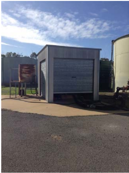
▲ Photograph 13: Former diesel AST and water tank to right of photograph.
