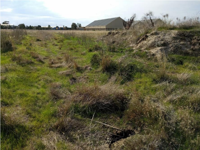
Photograph 5: Facing north, overflow drainage line from the dam (sample location SS07/SW03), showing it extending to the Deniliquin Freighter property.
