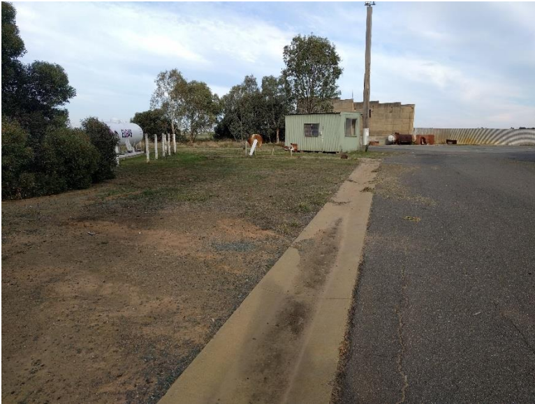
Photograph 1: Shallow drain on-site extending from the former AFFF use area towards a deeper drain
