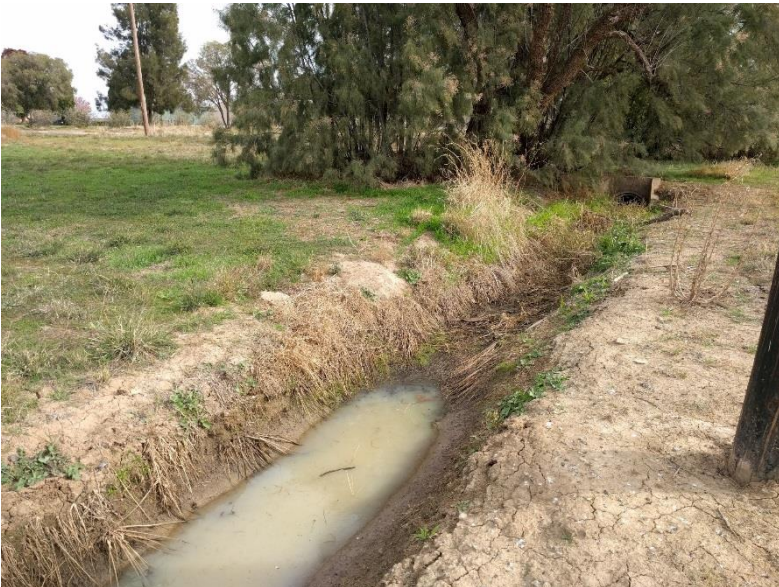
Photograph 6: Starting point of the eastern drainage line, believed to be the former drainage path from the site, showing an underground pipe as the starting point.
