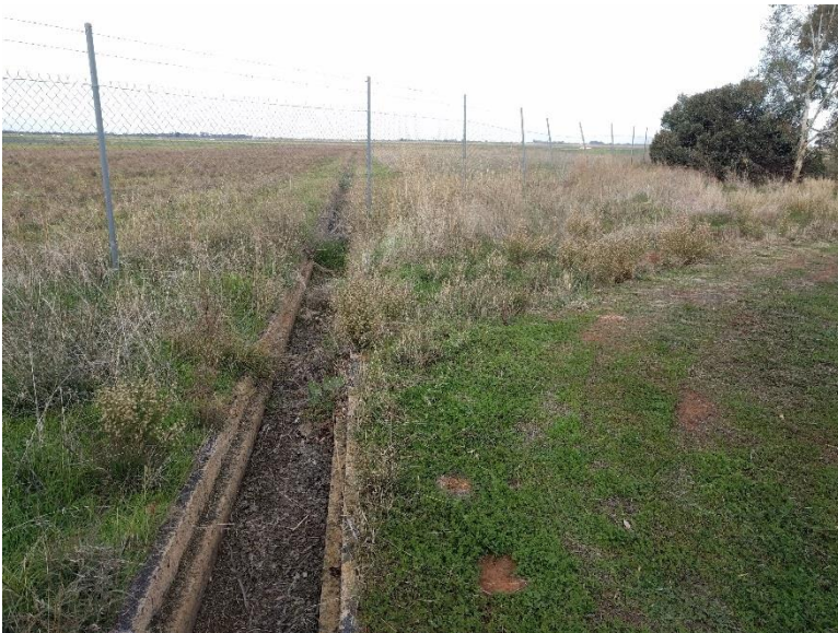
Photograph 2: Deep drainage channel on-site, extending onto the airport (south-east)
