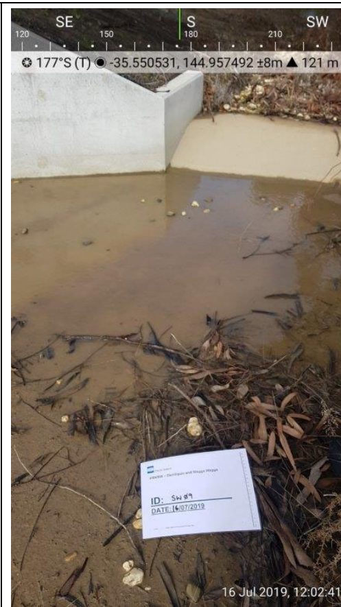
Photograph 2 Location SW09 within concrete lined drainage channel
