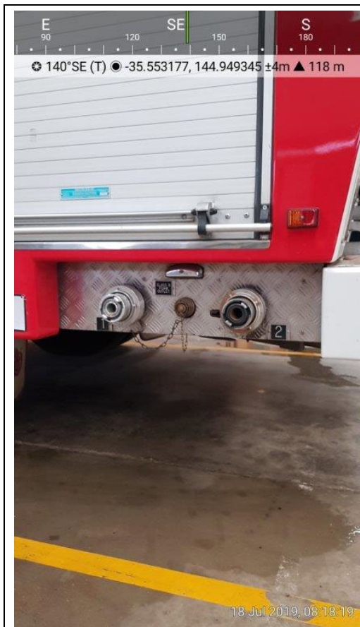
Photograph 5 Nearside sampling locations from the firetruck
