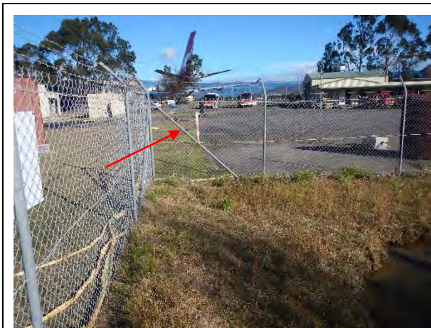
▲ Photograph 13: Facing west from the retention pond with the arrow showing a hose pipe entry where surface water is collected from the fire training ground.
