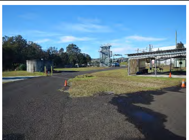
▲ Photograph 6: Facing south with the fire training structures.
